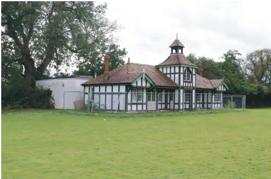
Plate 27. Oblique view of Sports Pavilion (Grade II Listed). Looking southwest.
