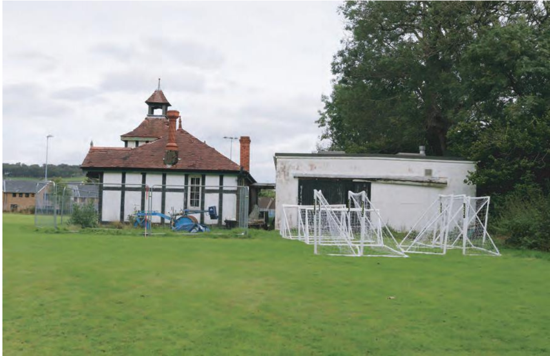
Plate 30. West facing elevation of Sports Pavilion (Grade II Listed). Looking east.
