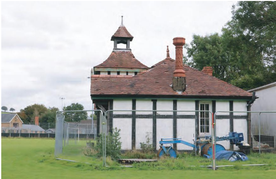
Plate 31. West facing elevation of Sports Pavilion (Grade II Listed). Looking east.
