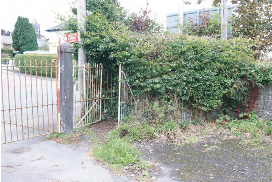
Plate 10. Iron 'Kissing' gate entrance into Playing Field. Looking northeast.
