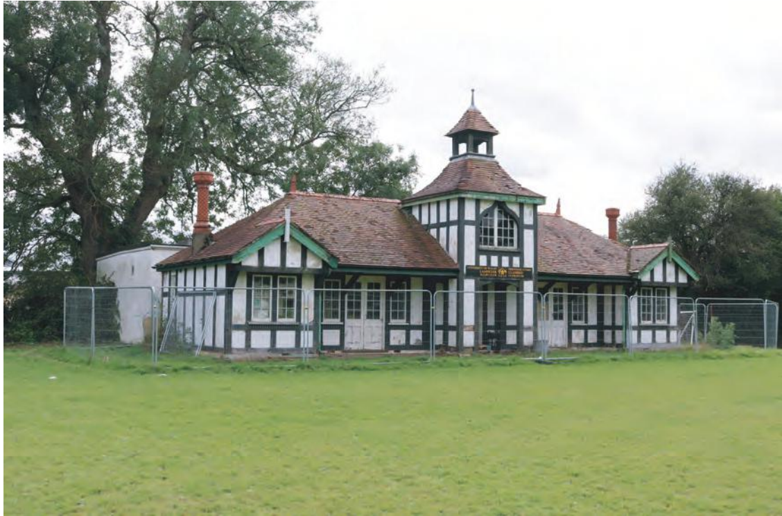
Plate 26. Oblique view of Sports Pavilion (Grade II Listed). Looking southwest.
