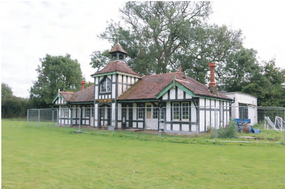
Plate 25. Oblique view of Sports Pavilion (Grade II Listed). Looking southeast.
