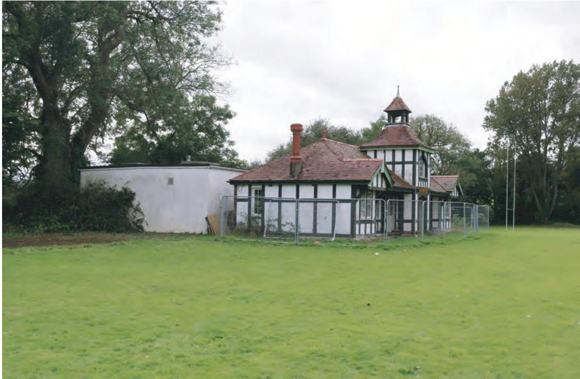
Plate 28. Oblique view of Sports Pavilion (Grade II Listed). Looking southwest.
