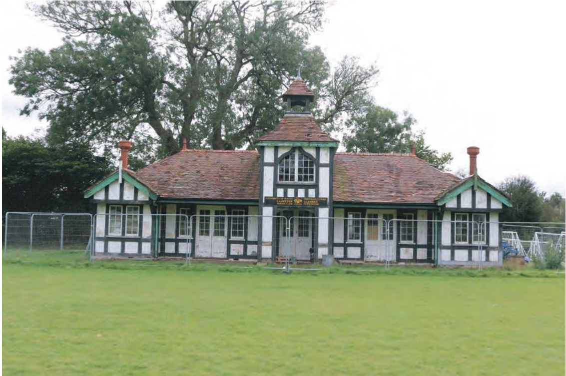
Plate 24. North facing elevation of Sports Pavilion (Grade II Listed). Looking south.
