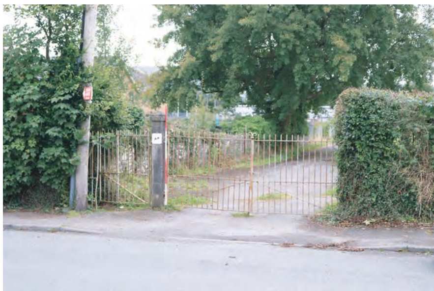
Plate 06. Iron entrance gates into Playing Field. Looking south.
