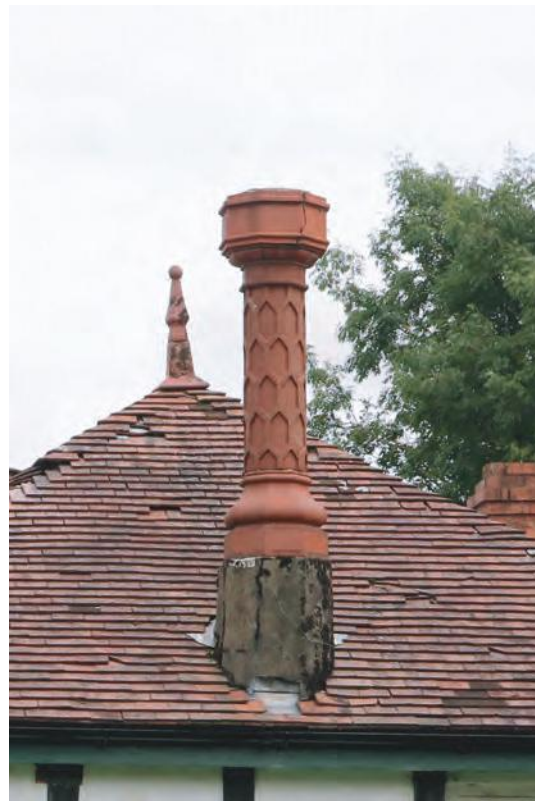
Plate 37. Detail of chimney of Sports Pavilion (Grade II Listed). Looking east.
