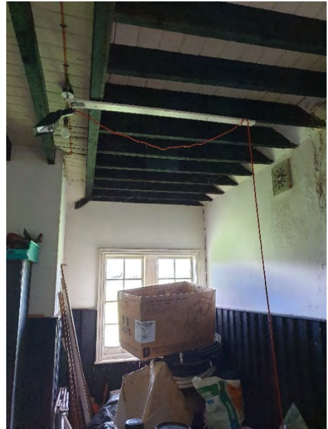
Photograph 18: Paired window on eastern gable block
