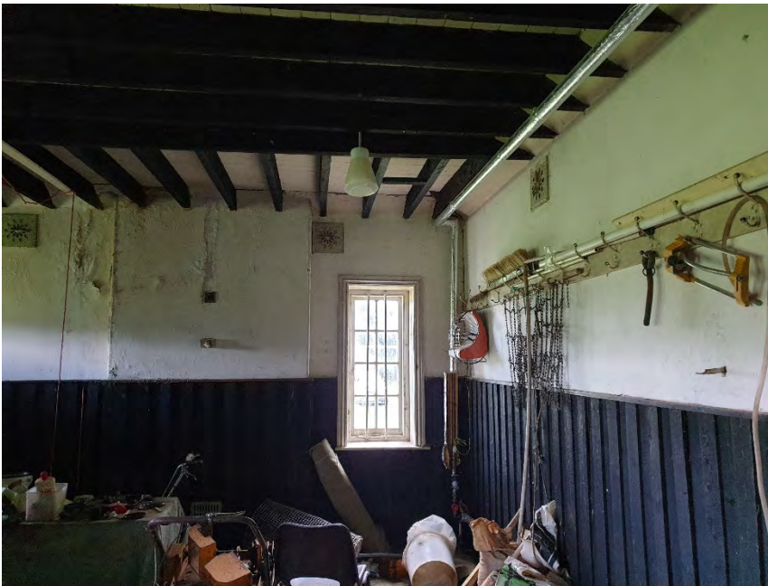
Photographs 30 to 31: Room to east of main entrance
