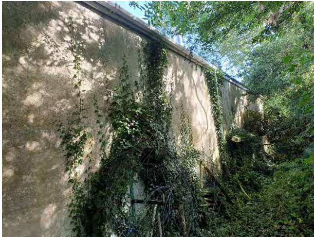
Photograph 22: Northern elevation (front)
