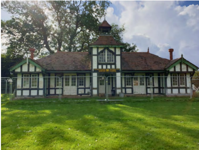
Photograph 3: Northern elevation (front)
