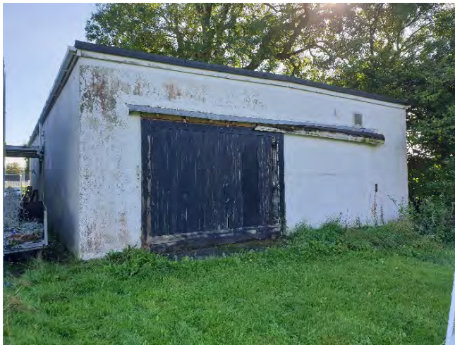
Photograph 19 and 20: Eastern elevation (side)
