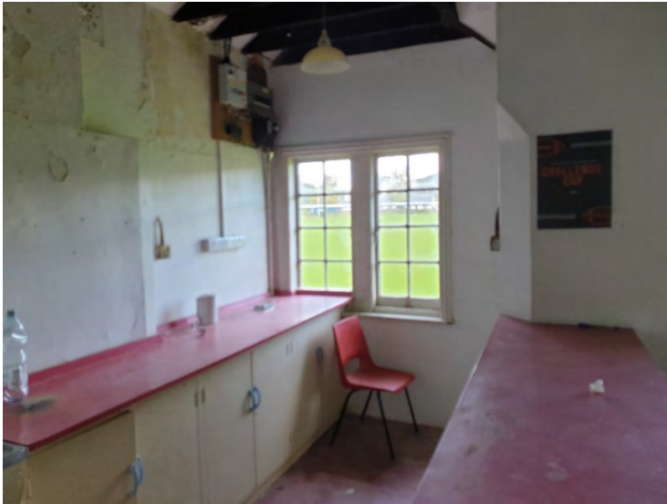
Photograph 17: Kitchen occupying the western gable block
