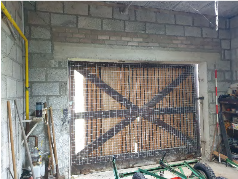
Photograph 26: Large sliding door in maintenance store
