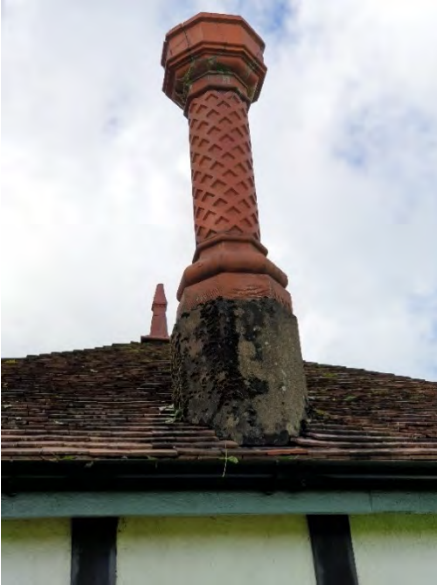
Photograph 7: Moulded terra cotta chimney
