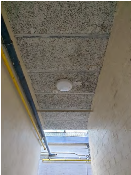
Photograph 23: Fire retardant ceiling above hall elevation (front)
