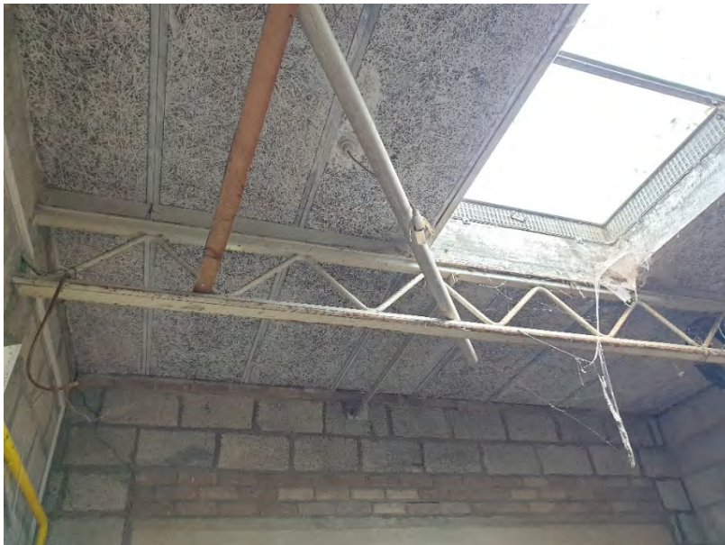
Photograph 25: Ceiling of maintenance store
