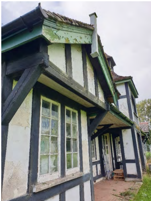
Photograph 11: Gabled blocks with paired windows either end of recessed entrance
