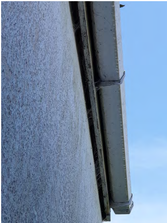
Gap behind lengths of wooden fascia – mostly covered in cobwebs
