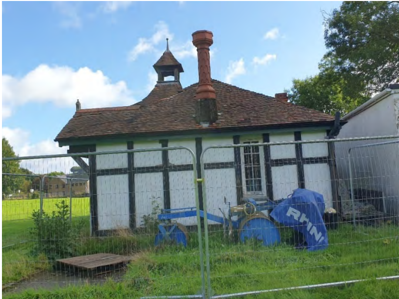
Photograph 2: Western elevation (side)
