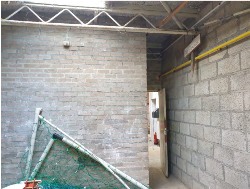
Photograph 24: Brick work and blockwork internal wall construction
