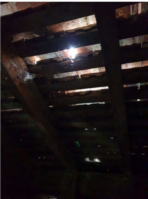
Photographs 12 to 14: Loft above western section of pavilion – timber truss construction, unlined roof with high levels of light ingress and fluctuating temperatures observed.
