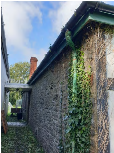
Photograph 4: Southern elevation (rear)
