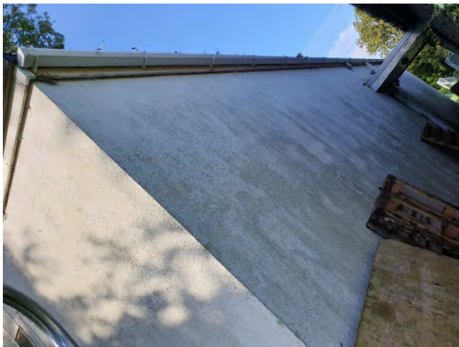
Photograph 21: Western elevation (side)
