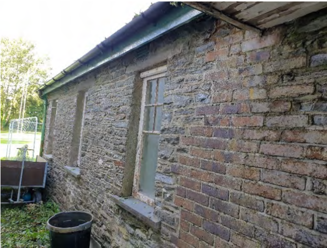
Photograph 8: Three multi-paned windows within stone built rear
