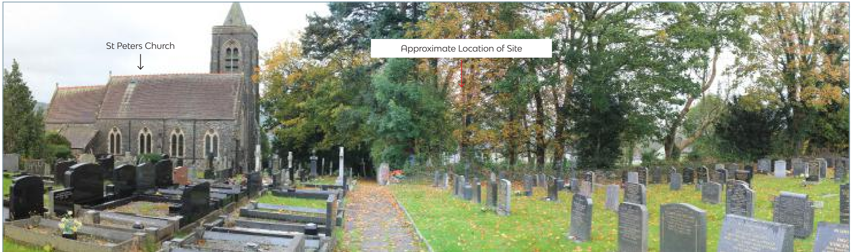
Photoviewpoint 6: Taken from St Peters Church graveyard at the end of the Aberaeron to Lampeter Trail looking towards the site
