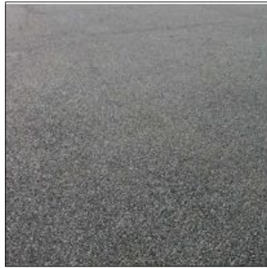
6 Tarmac beneath Aldi canopy
