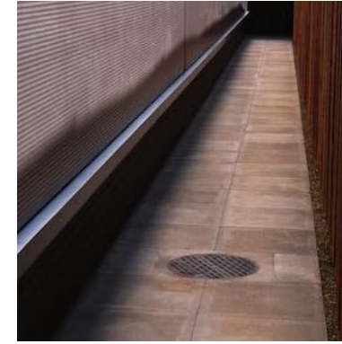
4 600 x 600mm concrete paving slabs to rear maintenance / escape area of Aldi. Colour grey
