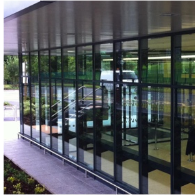
1 Shopfronts / window frames - polyester powder coated aluminium, colour - dark grey ral 7016 (anthracite)
