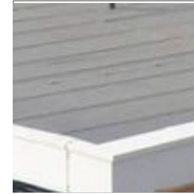
5 Roof - Kingspan 'Topdeck' KS1000/71/TD/ECOSAFE with composite membrane.
