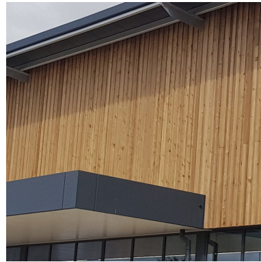
7 Wall - Timber rainscreen cladding.
