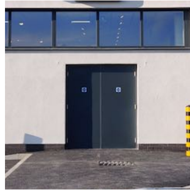
3 External escape doors and frames, steel polyester powder coated finish, colour - dark grey ral 7016 (anthracite)
