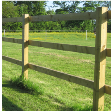
6 Timber Post and Rail Fence, 1200mm high.
