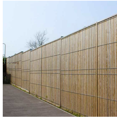
7 Plant Enclosure - Paladin Fence with timber inserts (To the south and west), 2400mm high.
