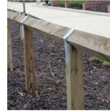
5 Timber Knee Rail with 100mm wide zinc straps
