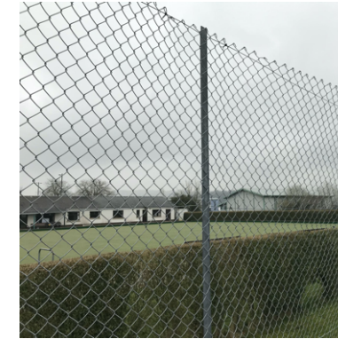
9 Existing chain link fence
