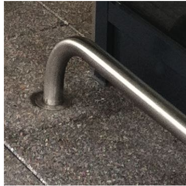
1 Aldi: Brushed stainless steel low level shopfront protection rails
