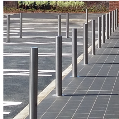
3 Aldi: Autopa Ltd stainless steel anti-ram bollards, 900mm high above ground, located to front of store between car park and public realm
