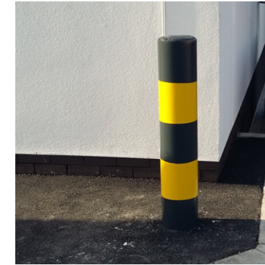
4 Aldi: Galvanised steel heavy duty bollard with concrete infill, painted black and yellow
