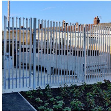
8 Palisade fencing, 2.5m high to external refrigeration plant enclosure. Finish - galvanised
