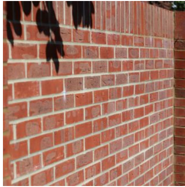
1 Red facing brickwork boundary wall
