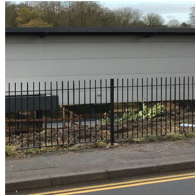
2 1.1m high metal railings around north and west site boundaries dividing site from the adjoining road and roundabout
