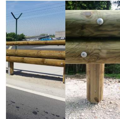
4 Timber-Steel Vehicle Restraint Barrier
